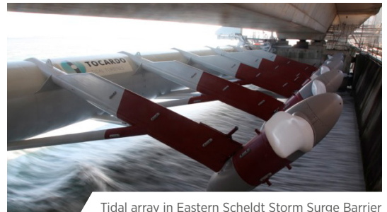
Tidal array in Eastern Scheldt Storm Surge Barrier
